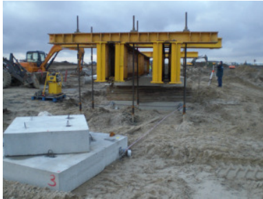
Load test for a bored pile
